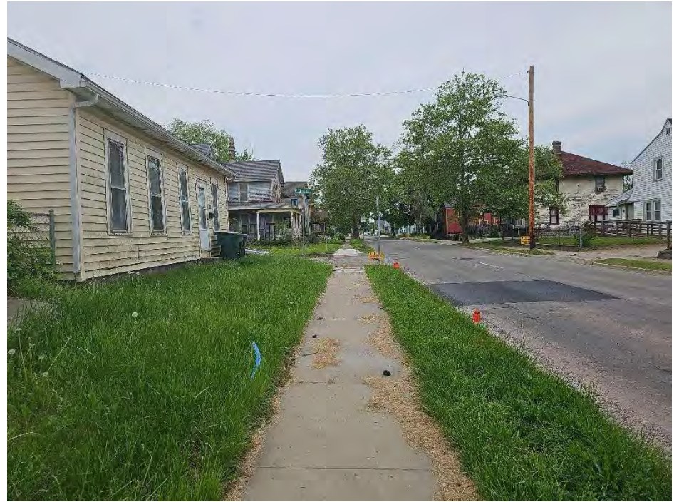
14. Looking west along the south side of EB SR 32/Jackson St.
