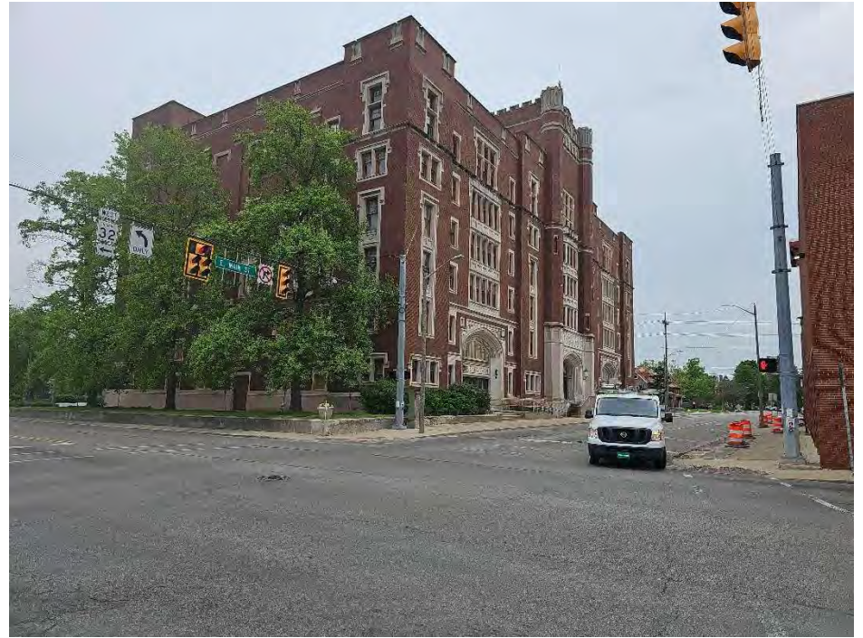
6. Looking northeast across the intersection of WB SR 32/Main St. and Madison St.
