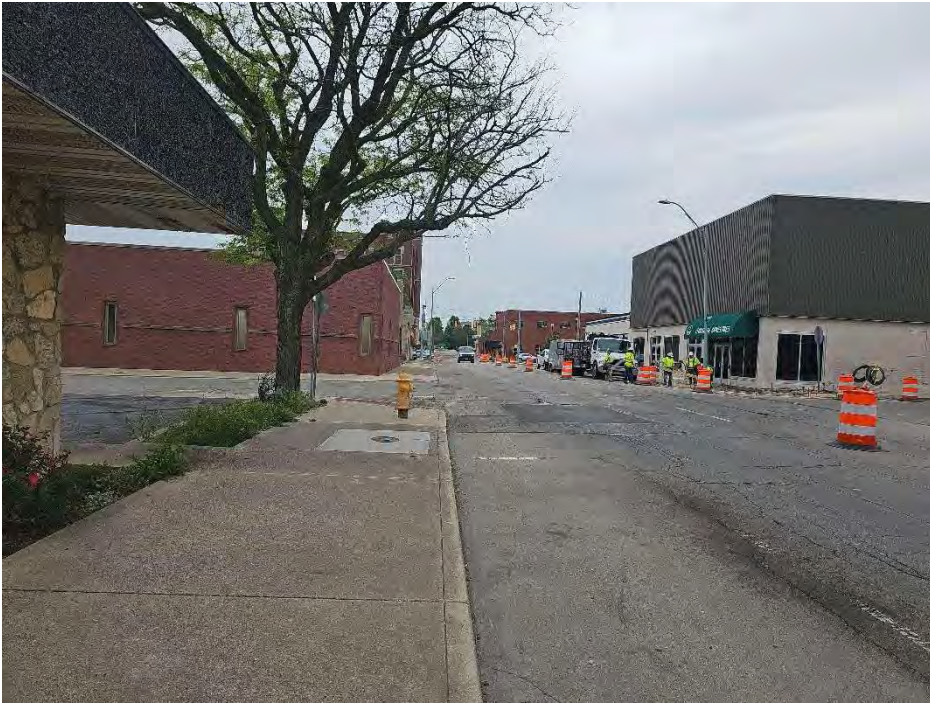
5. Looking east along the north side of WB SR 32/Main St.
