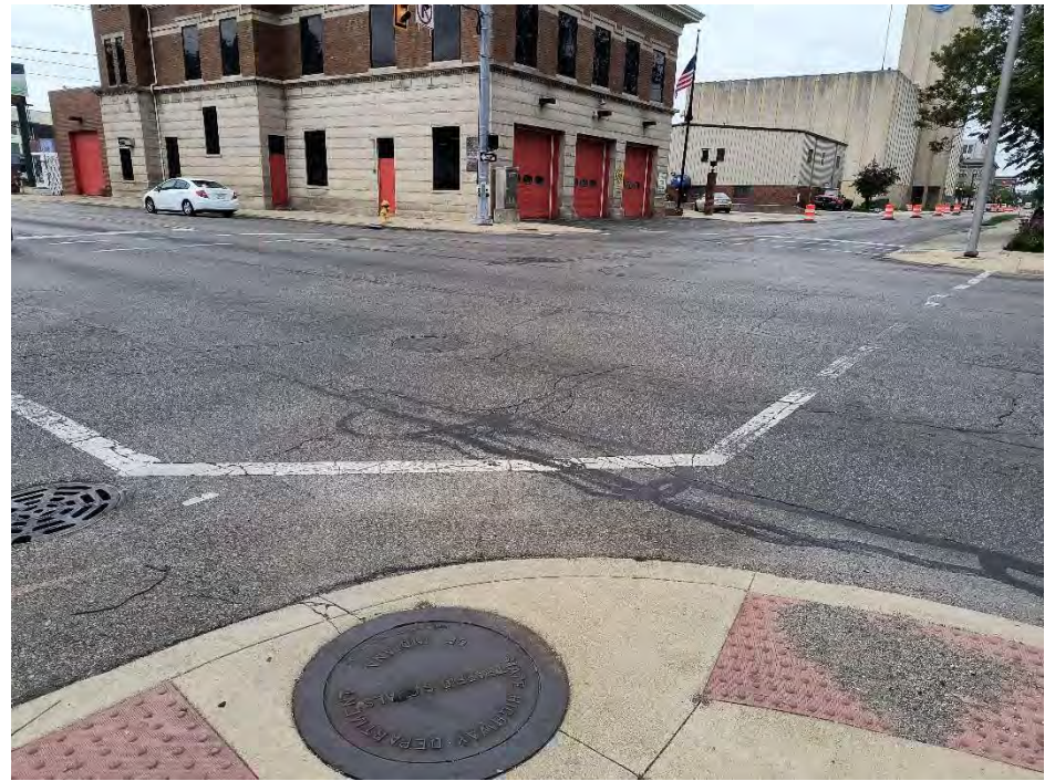
2. Looking southwest across intersection of EB SR 32/Jackson St. and Madison St. at Fire Station.
